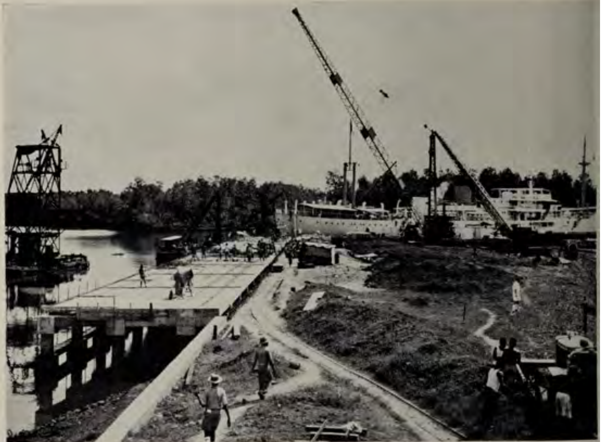
TIKO WHARF—CONSTRUCTION OF LIGHTER BERTHS
