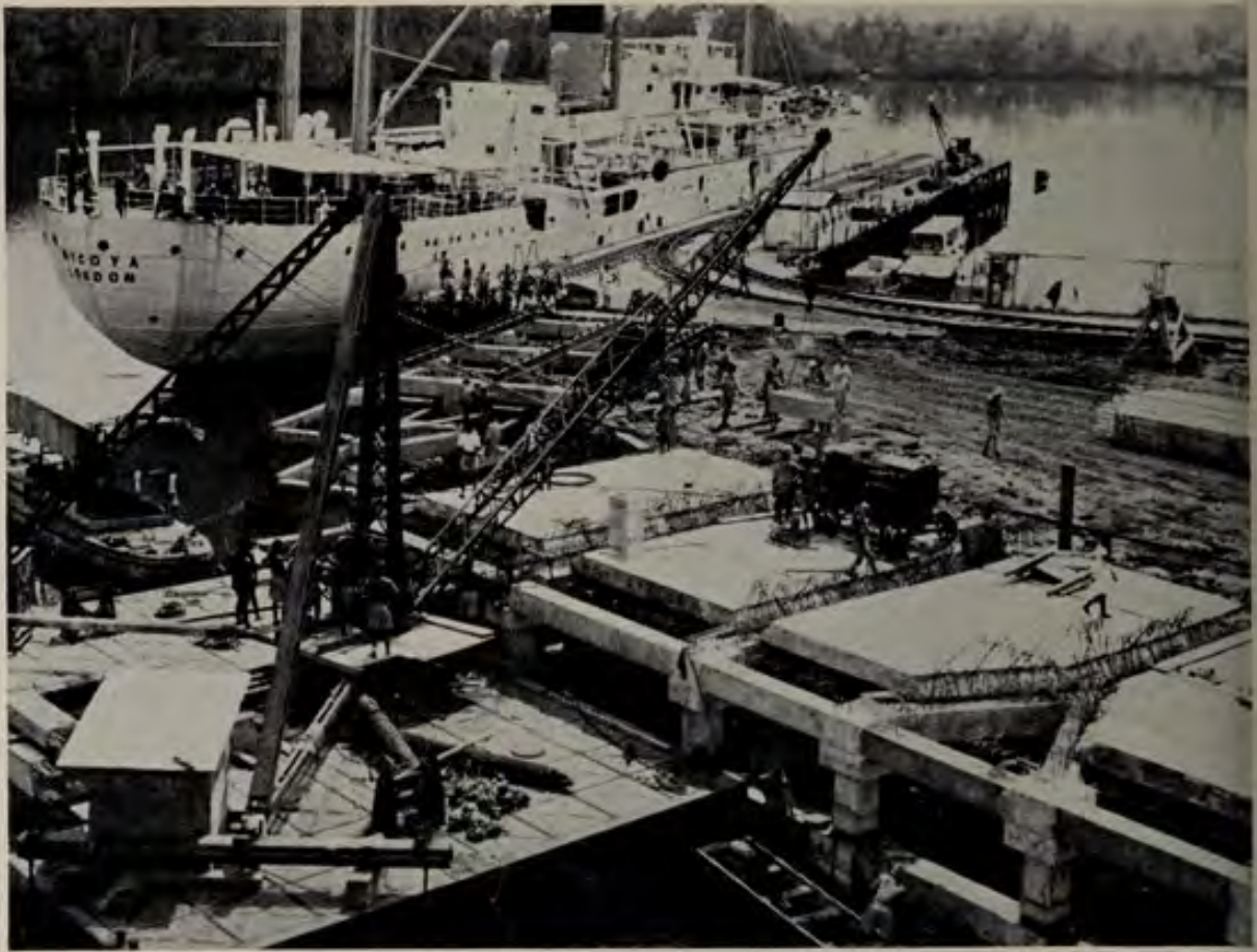
TIKO WHARF—CONSTRUCTION OF LIGHTER BERTHS
